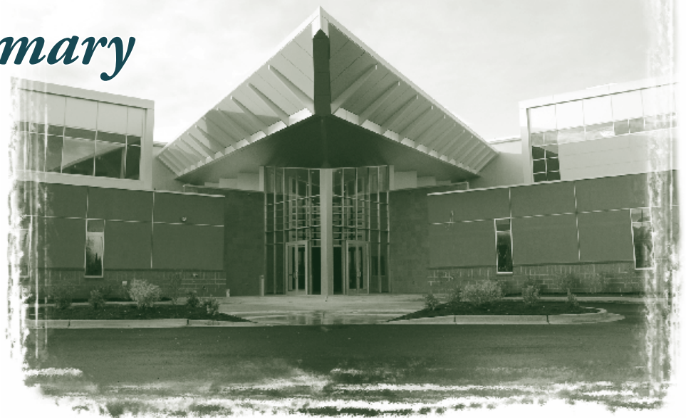
The new Alaska Psychiatric Institute in Anchorage.
