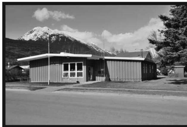
The Dahl Memorial Clinic in Skagway is located in picturesque Southeastern Alaska, and is accessible only by water or air. A new building is being planned.
